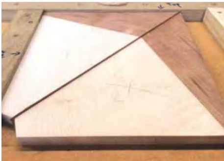
▲ Pic.17 I drew a rod of a quarter inside the jig to make sure that every quarter was exactly the same size. I did leave a few millimetres over-size to shoot down the doors when fitting them
